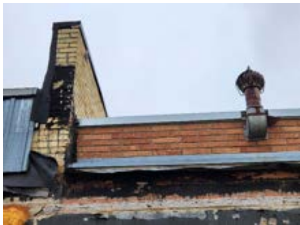
Top of wall conditions at demoed south wall and city hall north wall.
