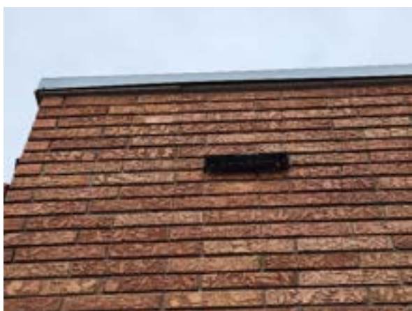
Existing roof scupper on city hall west wall.
