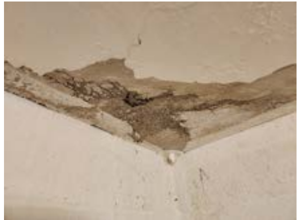
Ceiling of vault space in the lower level.
