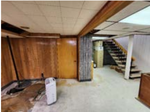
Existing sump pail serving the north half of the building.
