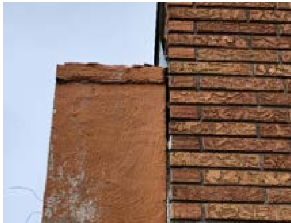
Gap in between the demoed south wall and city hall north wall
