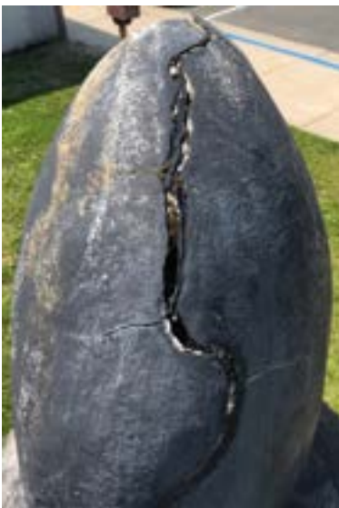
Figure 2 (Left). Large open crack spanning the length of the head.
