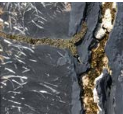
Figure 6 (Left). Detail of crack with old caulk and moss present.
