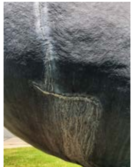
Figure 5 (Right). Crack exuding efflorescence, indicating water is moving through the cement but has no other egress.
