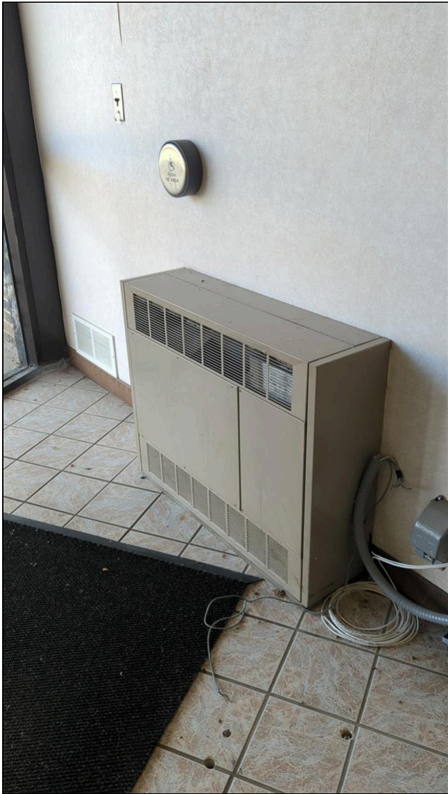
4.0 Item 5(Picture) entry vestibule
