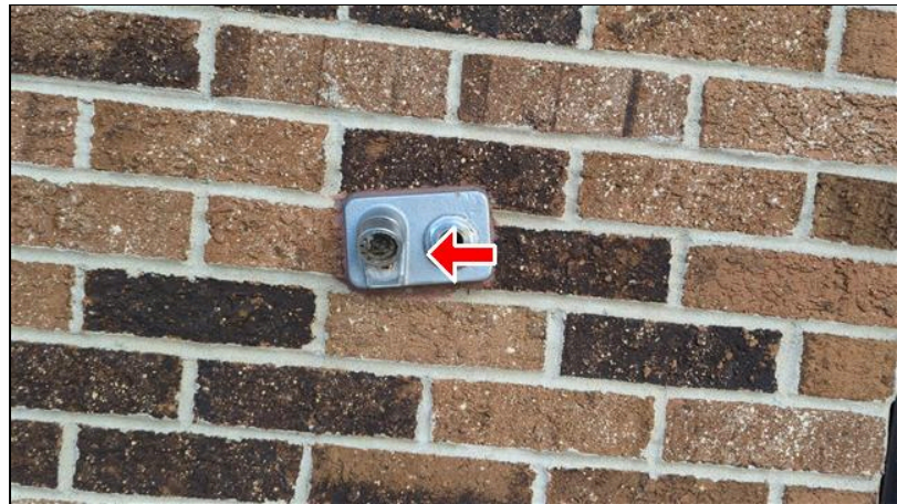
5.1 Item 2(Picture) back entry hose bib
