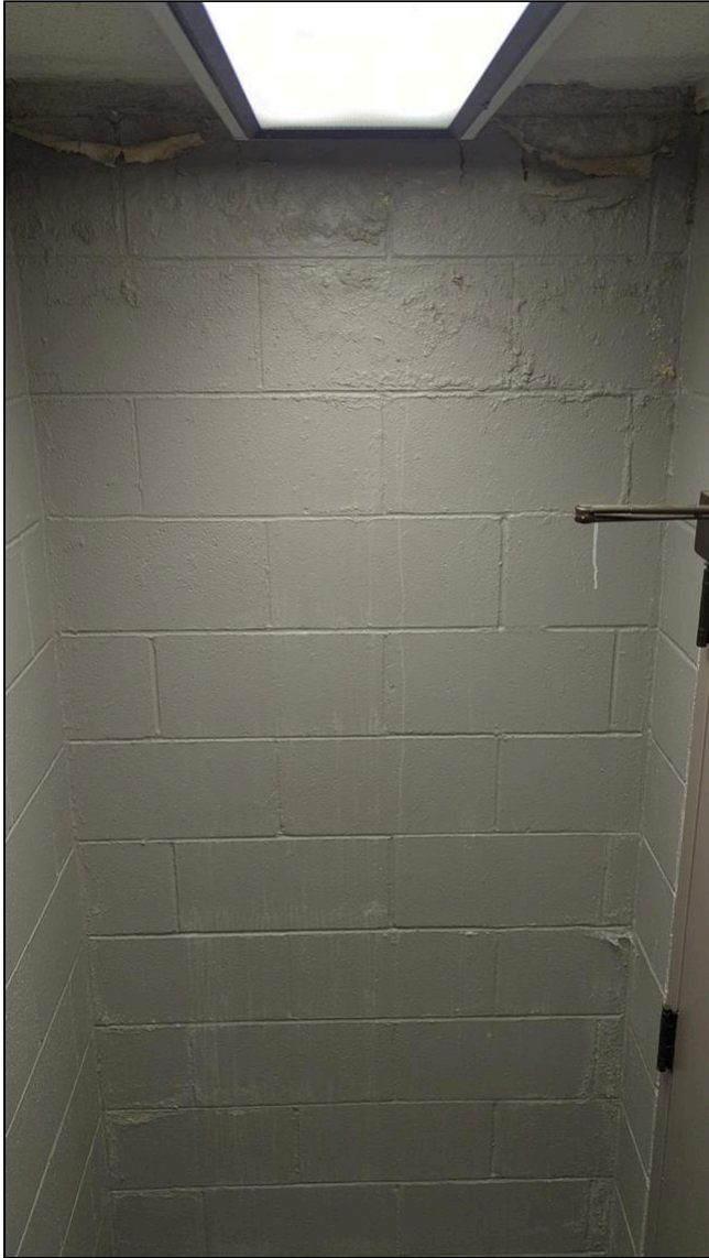
3.0 Item 11(Picture) south stairwell
