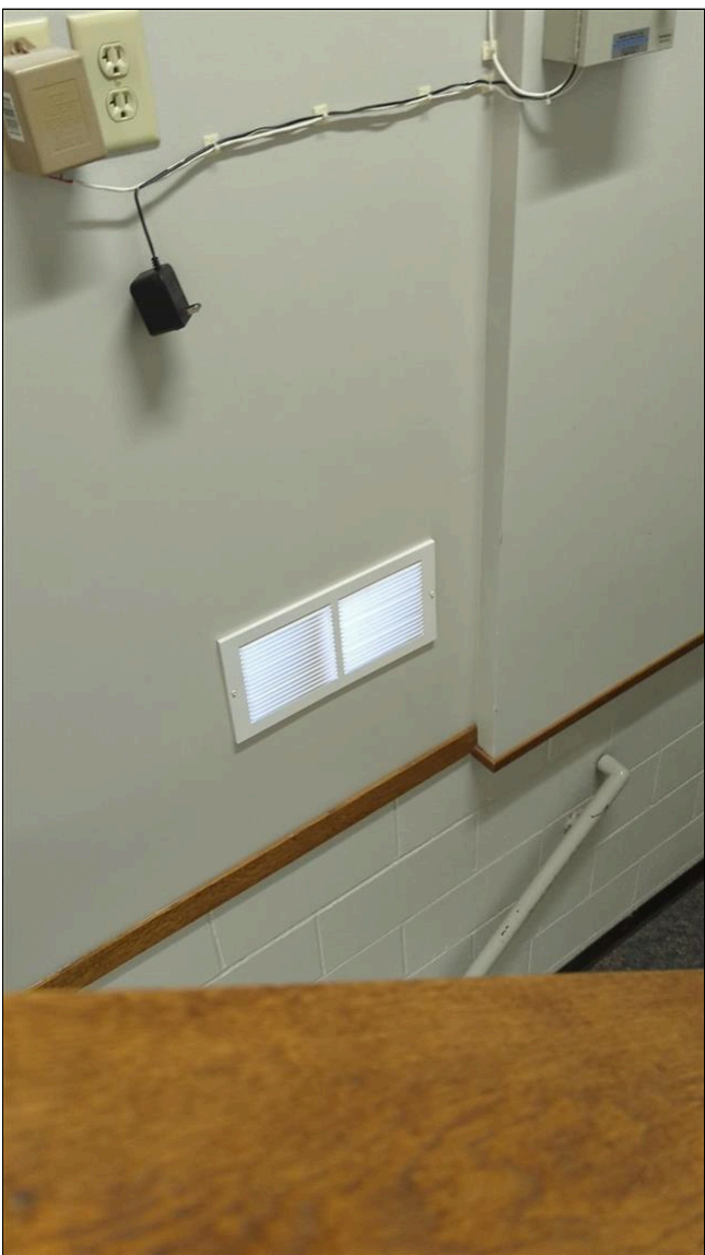
4.3 Item 2(Picture) retrofit return
