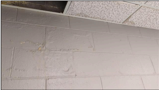
3.0 Item 9(Picture) ceiling/wall stains/peeling paint
