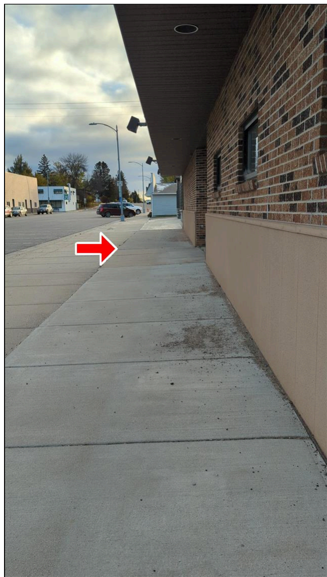
2.5 Item 1(Picture) low to negative pitch
