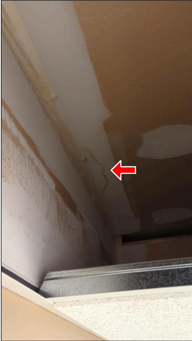
7.0 Item 11(Picture) Common wall with neighboring building
