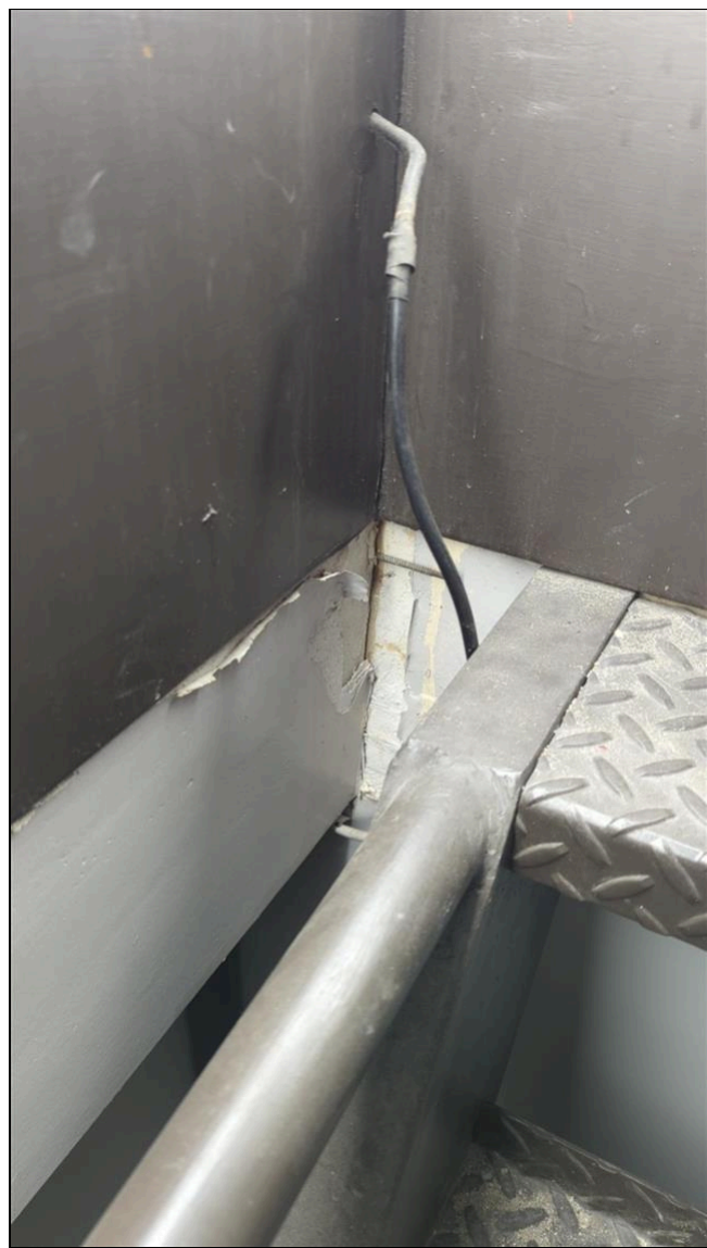
1.2 Item 1(Picture) inside roof access hatch
