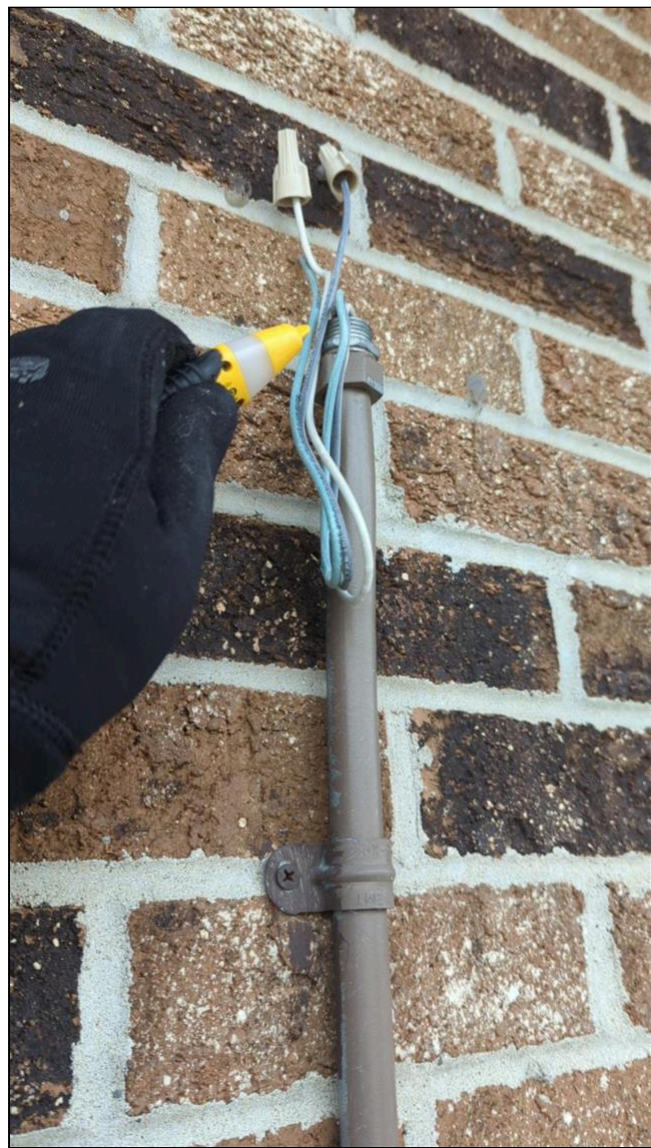
6.2 Item 1(Picture) W side of building
