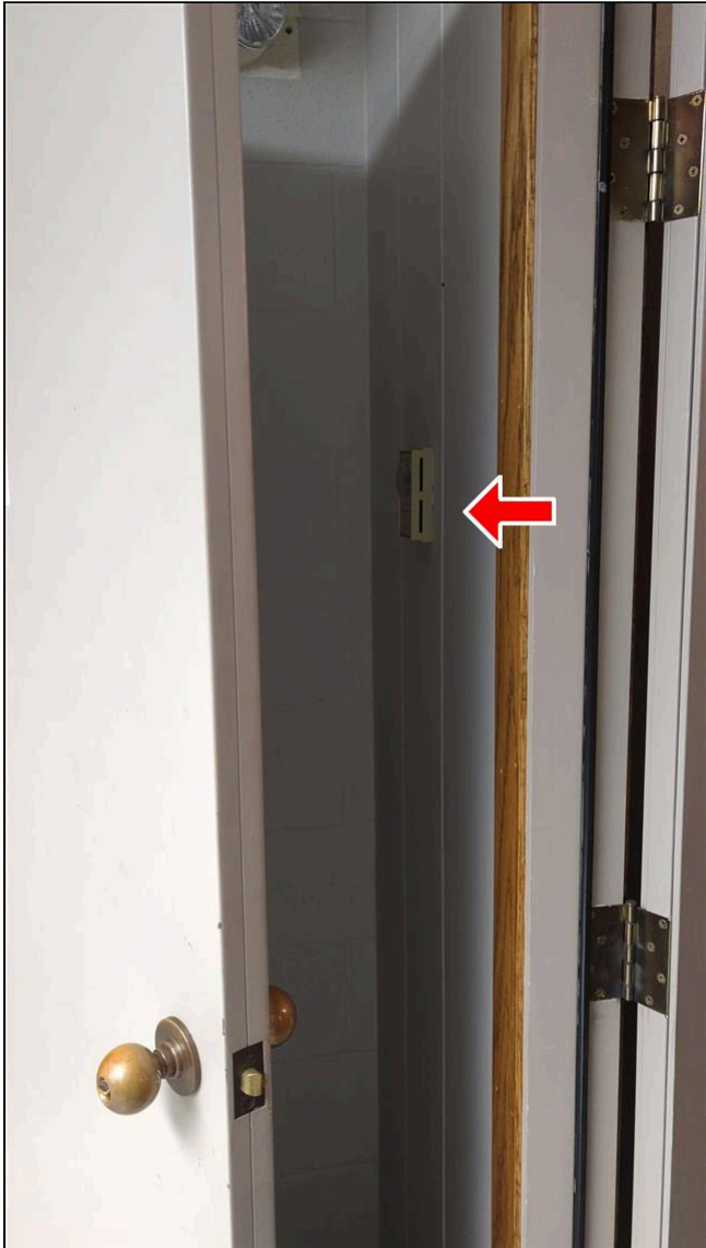
4.1 Item 11(Picture) basement
