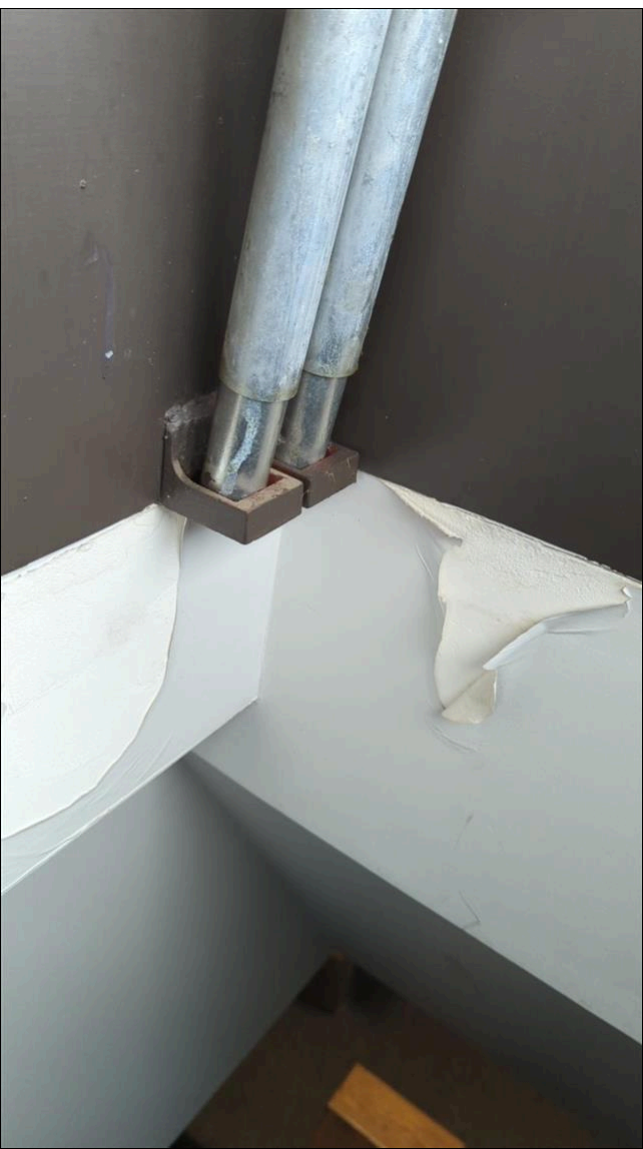
1.2 Item 2(Picture) inside roof access hatch
