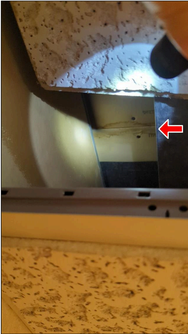
7.0 Item 6(Picture) above ceiling first floor men's room
