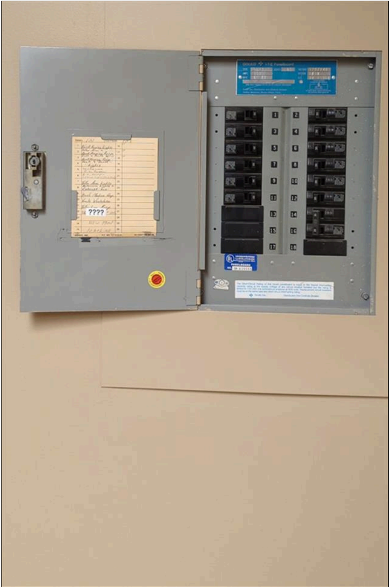
6.1 Item 5(Picture) near main floor restrooms 17 Summit Ave
