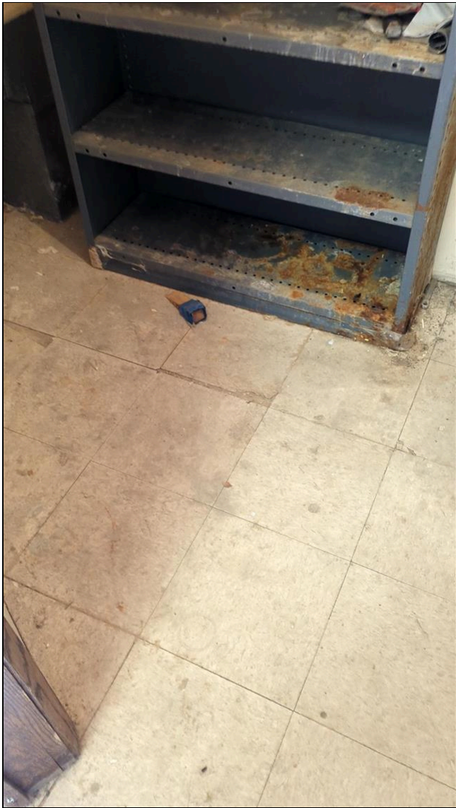
7.2 Item 1(Picture) janitor closet
