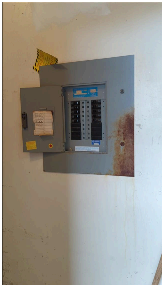
6.1 Item 1(Picture) janitor closet
