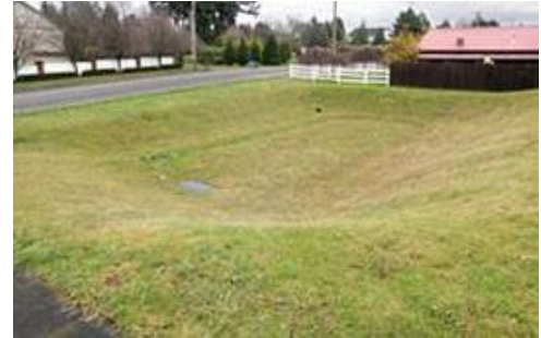
Example of an infiltration basin
