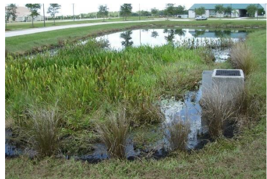
Example of a retention pond
