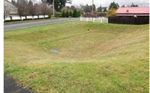
Example of an infiltration basin
