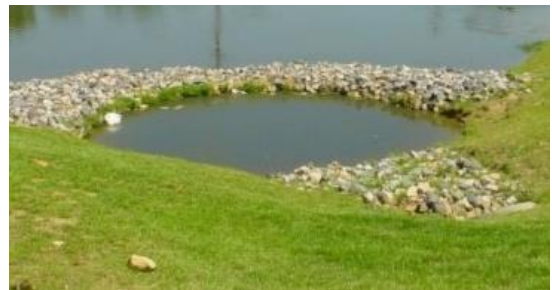
Example of a forebay
