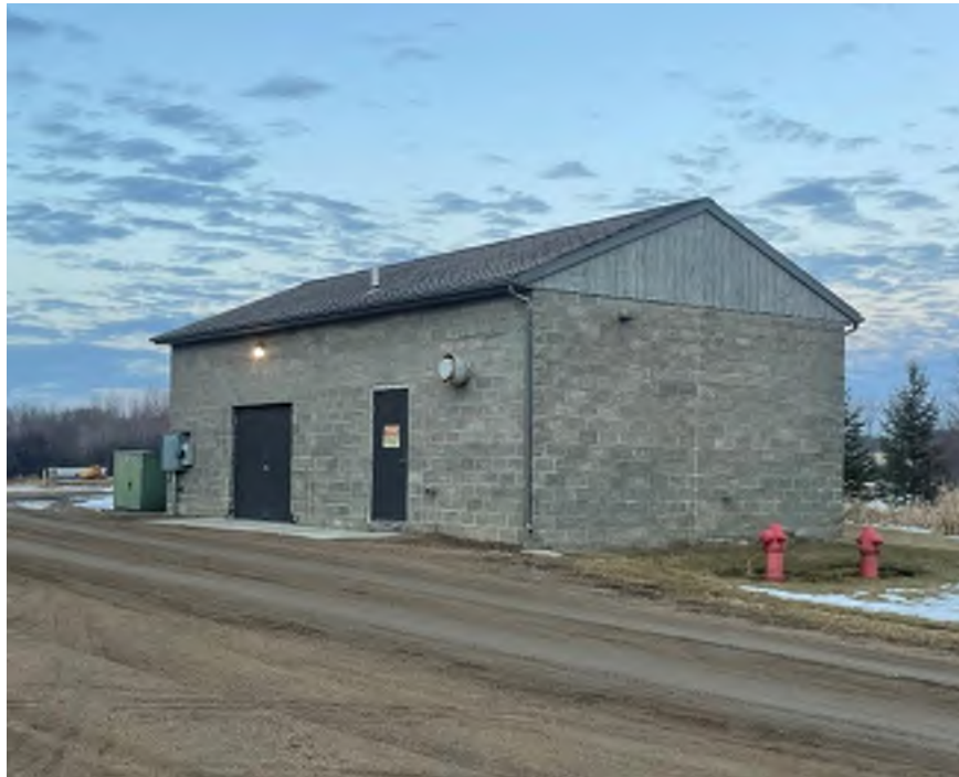
Figure 2-3 Existing Water Treatment Facility
