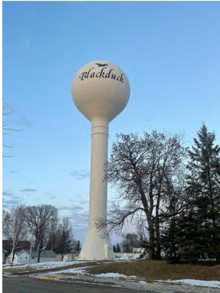
Figure 2-6 Elevated Water Storage Tank
